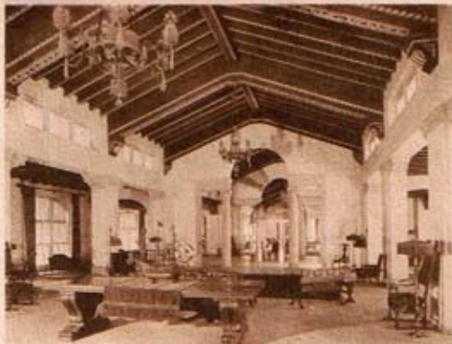
LOOKING THROUGH EAST LOUNGE AND PASSAGGIO TO WEST LOUNGE
