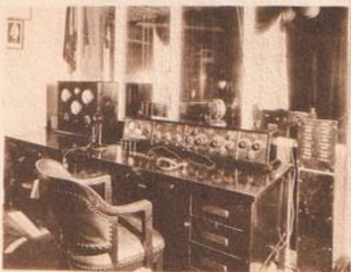
RADIO OPERATING ROOM - WEBH
