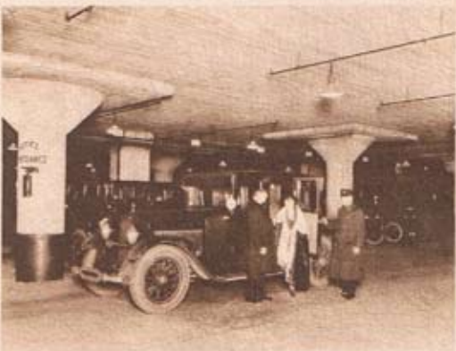
EDGEWATER BEACH HOTEL GARAGE ACCOMMODATING 200 CARS OF RESIDENT GUESTS. THE ONLY HOTEL IN CHICAGO OFFERING THIS SPECIAL SERVICE
