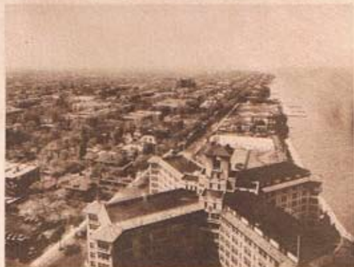
VIEW FROM ADDITION TOWER LOOKING NORTH
